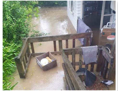
A flooded Visionwest property.
