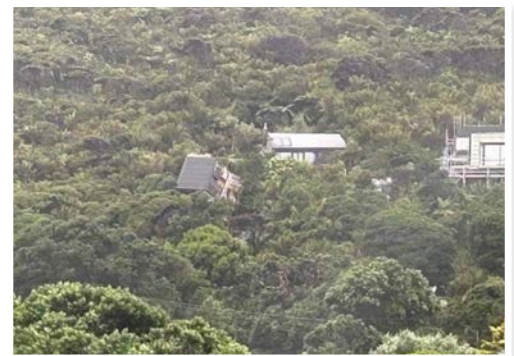
Landslip affected houses in West Auckland
